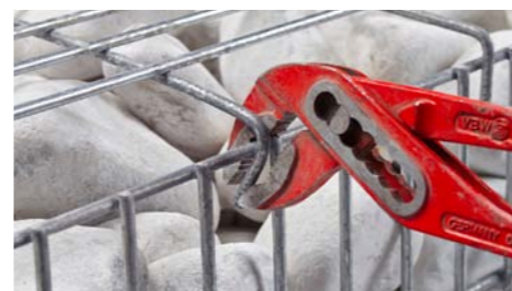
Tighten the hooks with pliers.
